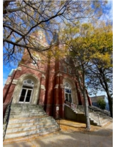
York County Commissioners have approved up to $1.5 million in funding to help renovate the former St. Andre Church on Bacon Street in Biddeford into My Place Teen Center. The center still has to raise some funds and in-kind support for the project. It is projected to open in 2023 and serve kids 10-18 from around the region. Tammy Wells Photo
